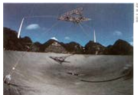
The Arecibo radio/radar observatory in Puerto Rico. The hemispherical reflecting dish is surmounted by the feed arms, which are supported by three large obelisks, two of which are seen distorted in the lower picture, taken with a fish-eye lens at the level of the panels that make up the dish. Courtesy of the National Astronomy and Ionosphere Center, Cornell University.
