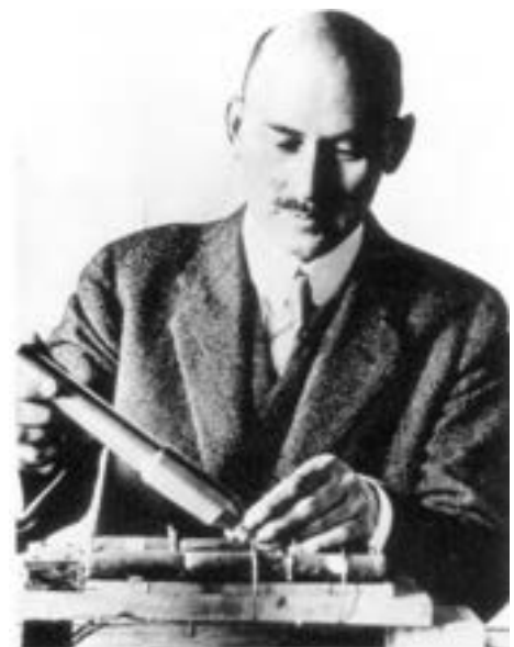
Goddard at age thirty-three, fitting a steel combustion chamber for a small solid-fuel rocket to a test bed. Courtesy Goddard Library, Clark University.
