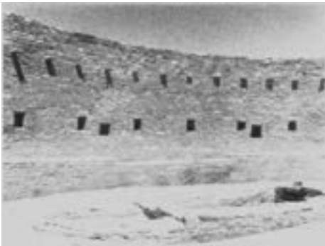
Interior of Casa Rinconada, showing six higher and two lower niches.
