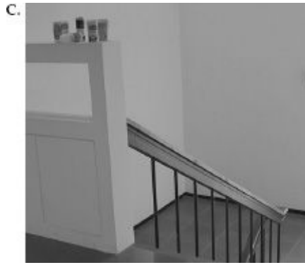
FIGURE 1.5. Accidental Affordances Can Become Strong Signifiers. This wall, at the Industrial Design department of KAIST, in Korea, provides an anti-affordance, preventing people from falling down the stair shaft. Its top is flat, an accidental by-product of the design. But flat surfaces afford support, and as soon as one person discovers it can be used to dispose of empty drink containers, the discarded container becomes a signifier, telling others that it is permissible to discard their items there. (Photographs by the author.)
