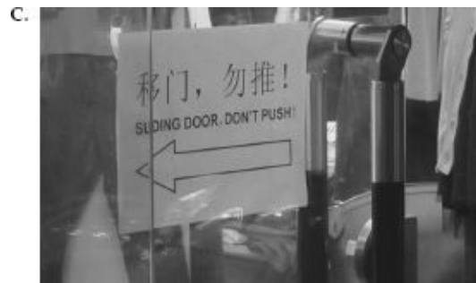
FIGURE 1.3. Sliding Doors: Seldom Done Well. Sliding doors are seldom signified properly. The top two photographs show the sliding door to the toilet on an Amtrak train in the United States. The handle clearly signifies “pull,” but in fact, it needs to be rotated and the door slid to the right. The owner of the store in Shanghai, China, Photo C, solved the problem with a sign. “DON’T PUSH!” it says, in both English and Chinese. Amtrak’s toilet door could have used a similar kind of sign. (Photographs by the author.)
