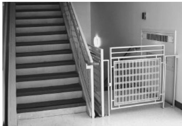
FIGURE 4.7. A Lockout Forcing Function for Fire Exit. The gate, placed at the ground floor of stairways, prevents people who might be rushing down the stairs to escape a fire from continuing into the basement areas, where they might get trapped.
