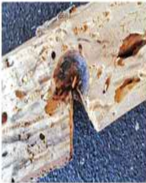
Repeat until you've chopped out the completed notch.
