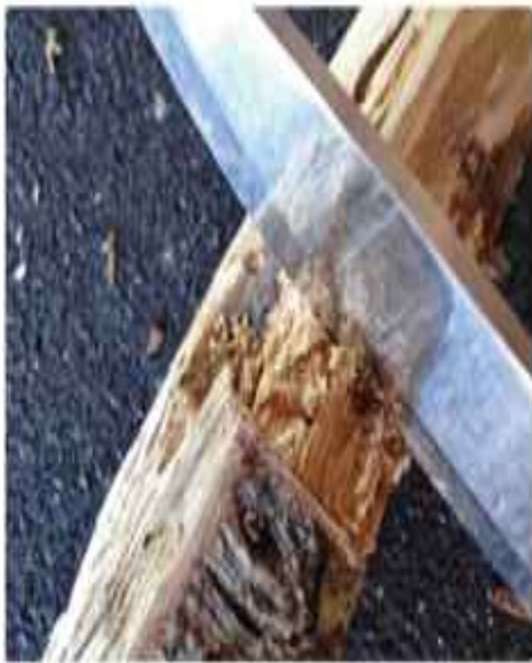
Make a \frac{1}{2} "- \frac{1}{4} " cut down either side of the notch with your blade, then pop that small section out.
